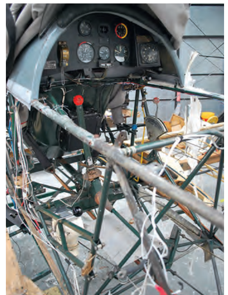
The fuselage tubing will need all the paint stripping from it and a new dope-proof anti-corrosion finish applied.
