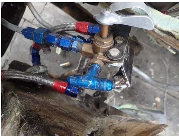
Fig. 1. This picture shows the return tee fitting as found on the aircraft involved in the accident; unused (return) fuel must be returned to the fuel tank where it has the opportunity to release any vapour bubbles that may have formed and can be cooled.
